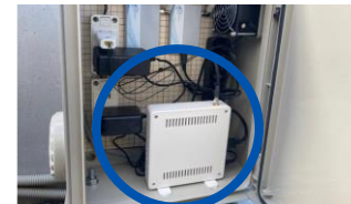
Demand control (centralized controller)
