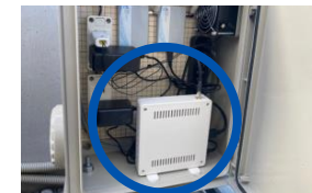
Demand control (centralized controller)
