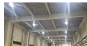
Installing LED based on green lease agreements
