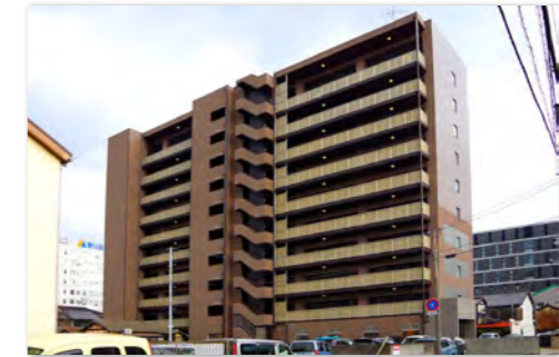
R-60 RESIDIA Okayama-Ekimae (Completed a large-scale repair in FP01-2017)
